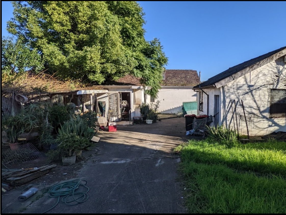
Figure 18. Rear view of the dwelling and garage shed within the property on No. 21 Ellis Street.
