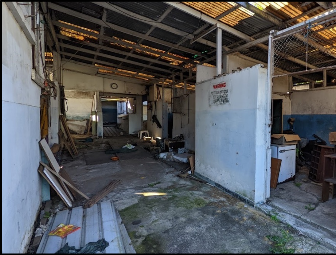
Figure 16. Inside of the stables within the property on No. 21 Ellis Street.
