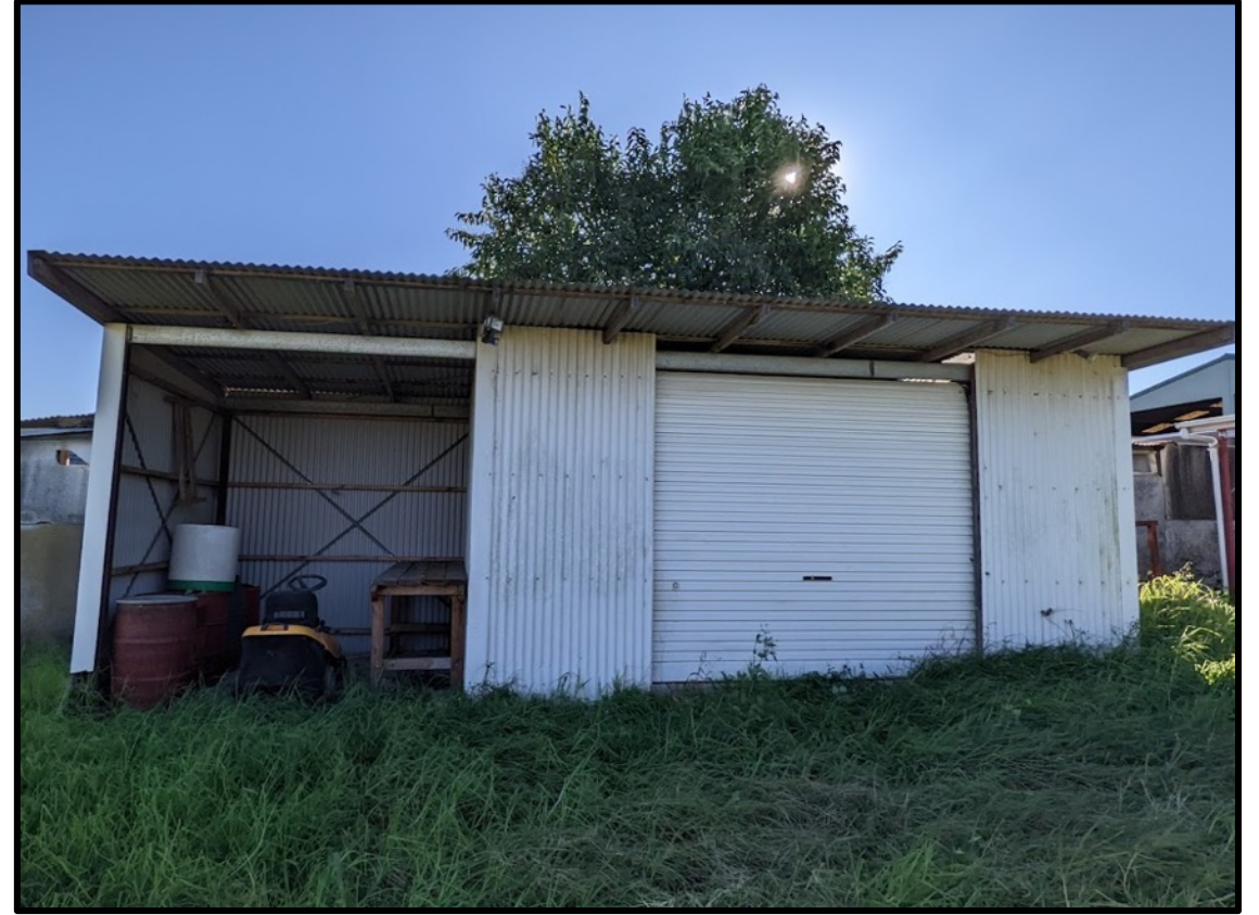
Figure 21. Metal shed within the eastern portion of the property at No. 23 Ellis Street.
