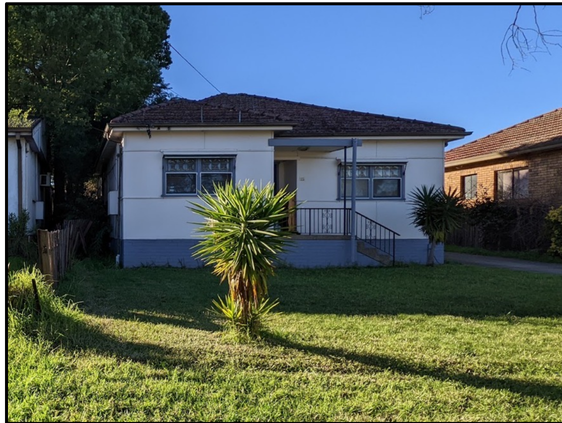
Figure 9. Front view of the fibrocement clad dwelling within the property on No. 23 Ellis Street.
