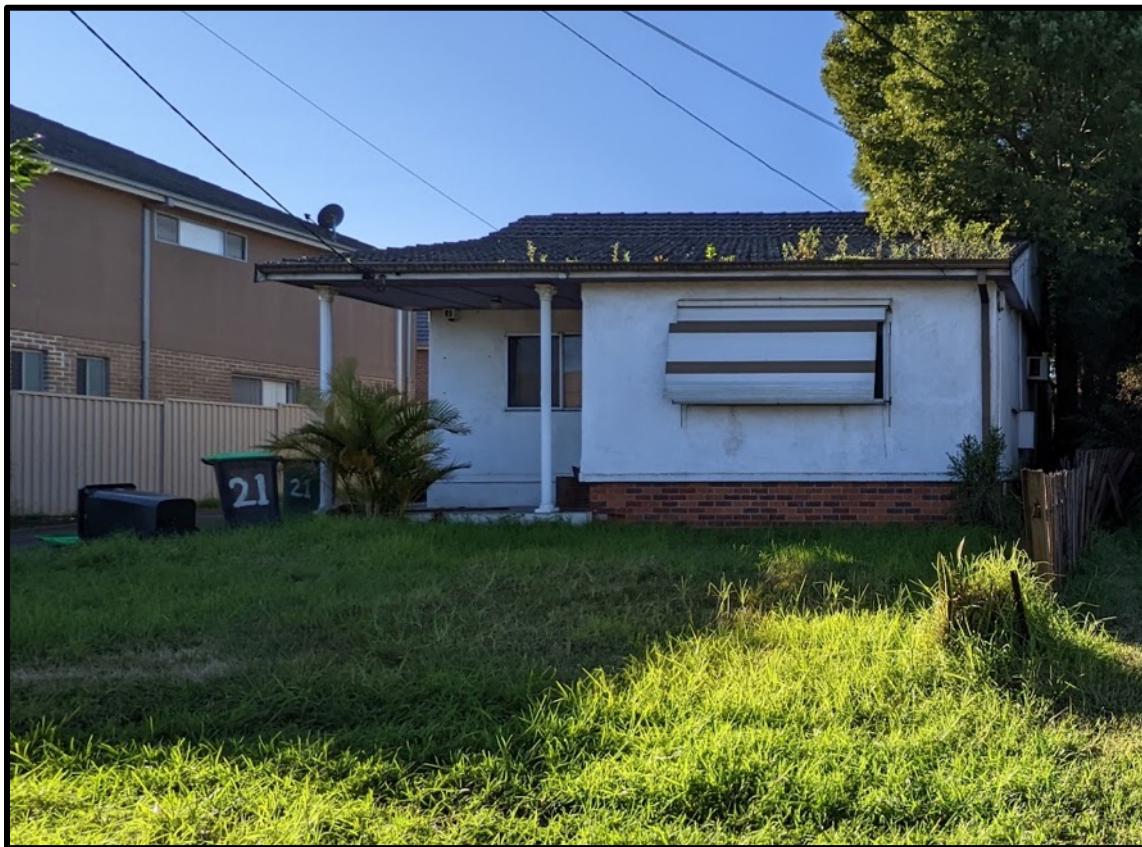
Figure 8. Front view of the rendered brick dwelling within the property on No. 21 Ellis Street.
