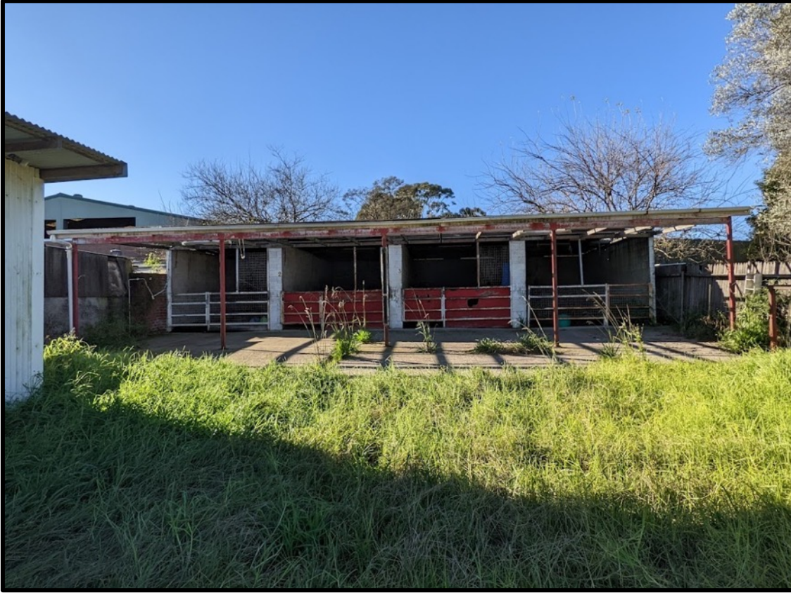
Figure 20. The clad stables and concrete slab with the eastern portion of the property on No. 23 Ellis Street.
